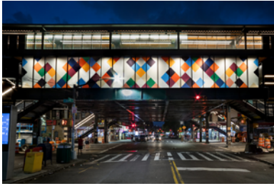
Perasma II , 2018, 8.5 x 66 foot frieze, 21 panels, laminated glass, East glass façade, MTA 30 th Street Station, Astoria, Queens
